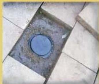
Installation under pavers
